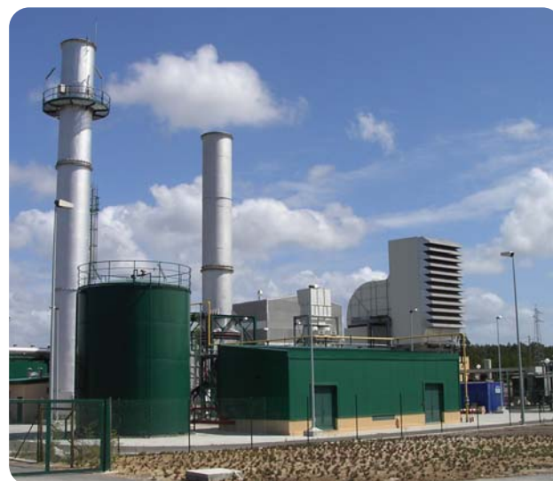
Carrigo Cogeneration plant
