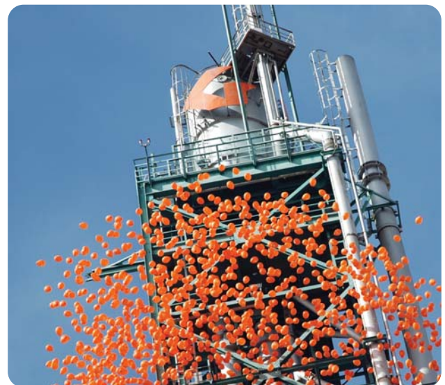
Galp Tower - Parque Expo
